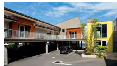
Constructors Hawaii's project at 3470 Waiialae Ave.
