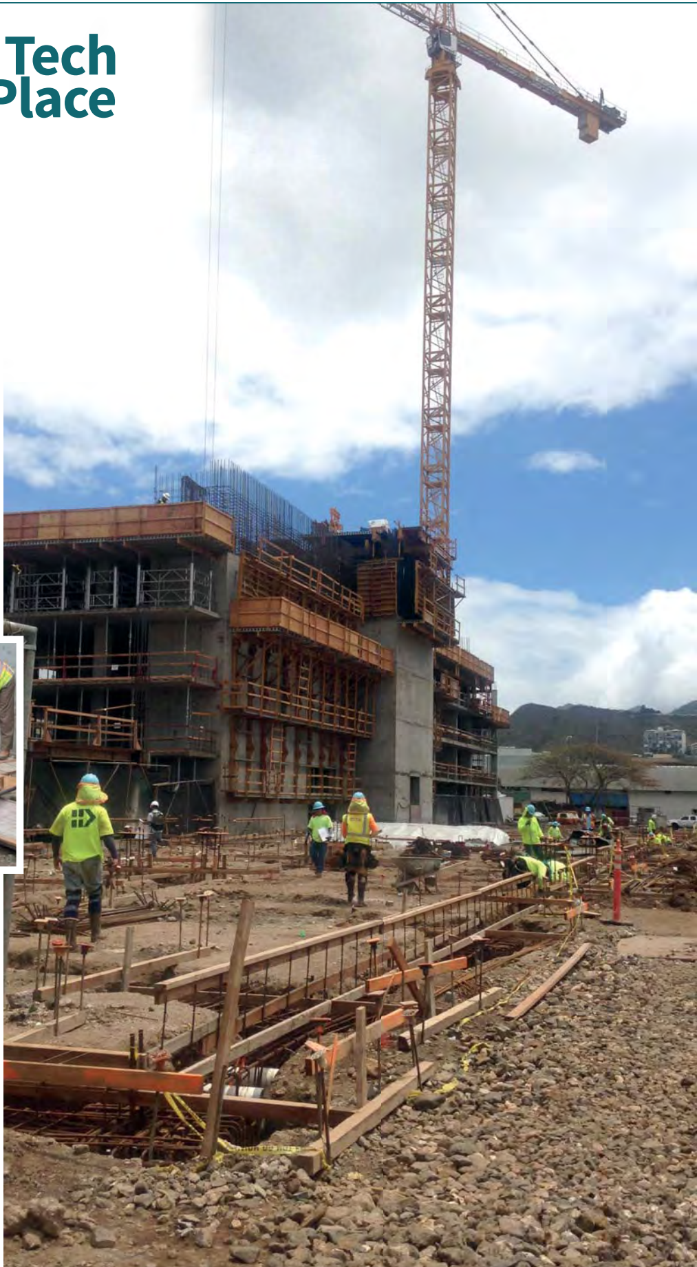
Tower crane at Keauhou Place jobsite
