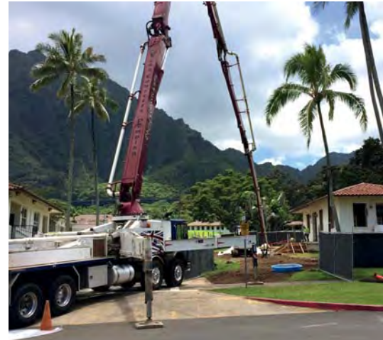
Paradigm Construction crews at work at Windward Community College.
