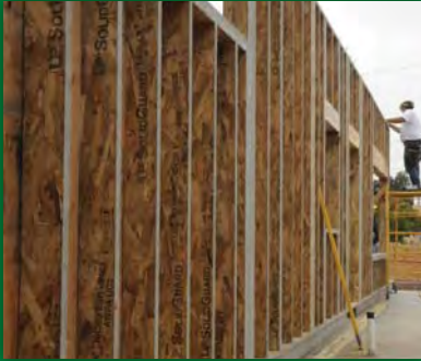
LSL WALL PANELS @ HOSPICE, KAMUELA
