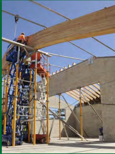
GLULAMS @ KEAUKAHA ELEMENTARY SCHOOL
