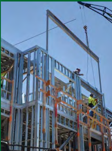
STEEL FRAMING @ KA MALANAI, KAILUA
