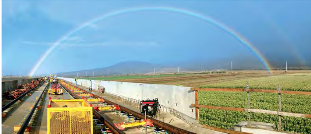
The rail along the guideway by Farrington Highway in West Oahu
