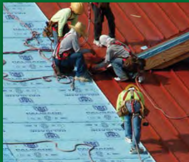
CUSTOM METAL ROOFING
