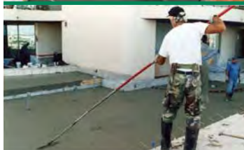
Moisture resistant and easy to pump, place and finish, Isle CellCrete was utilized to repair Harbor Court's 12th floor recreation deck planters.
