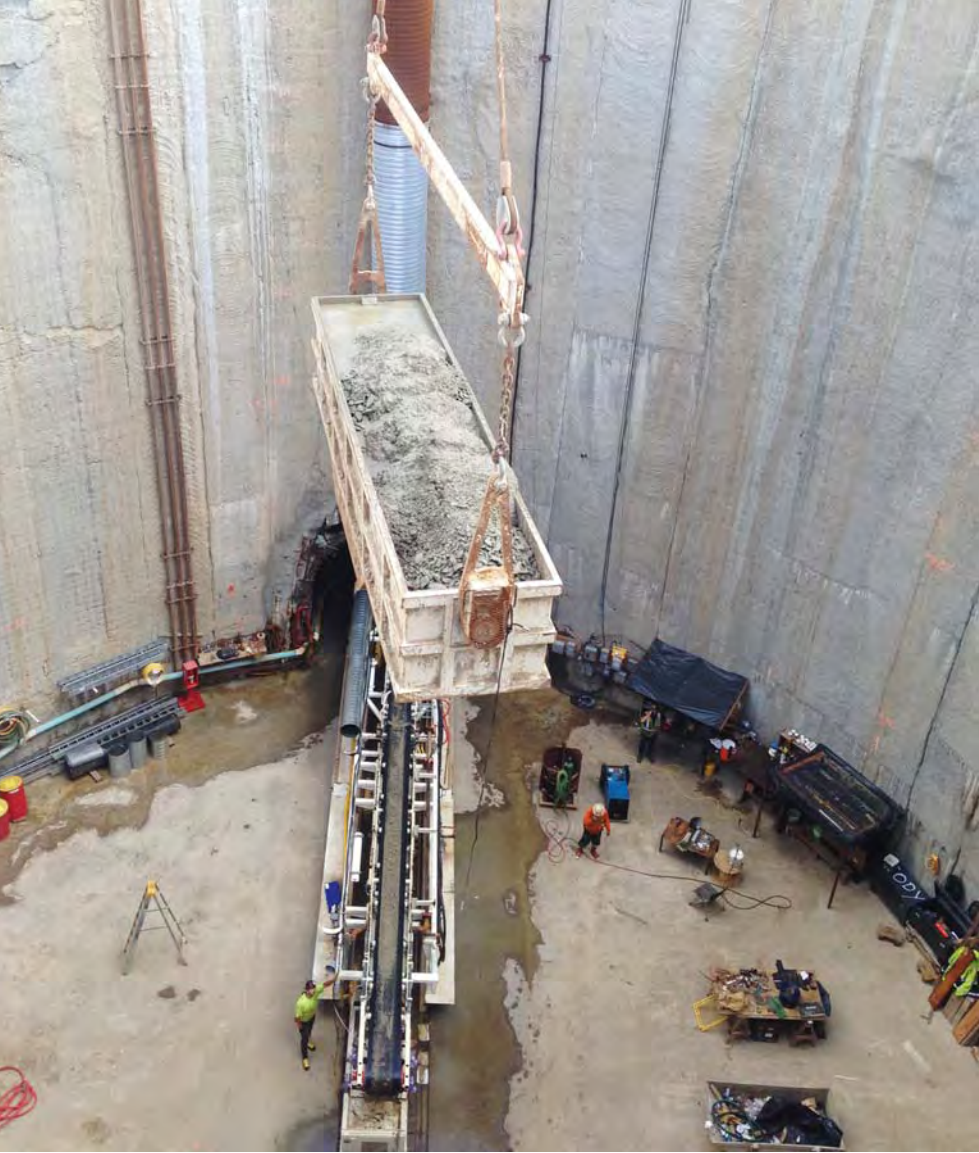
Muck removal at the City and County of Honolulu's Kaneohe Kailua Gravity Sewer Tunnel. PHOTO COURTESY CITY & COUNTY OF HONOLULU
