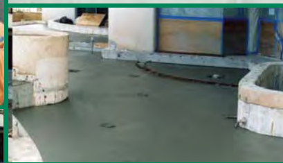
Moisture resistant and easy to pump, place and finish, Isle CellCrete was utilized to repair Harbor Court's 12th floor recreation deck planters.
