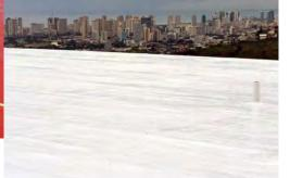
urethane fluid applied coating combines a polyuria base coat with a high solids silicone topcoat. Combining the fire retardant, durability and strength of an aromatic urethane with the UV and water resistance of silicone, this system extends the life of a roof system and withstands ponding water. www.allweathersurfaces.com
