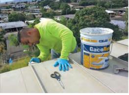
A Murakami Roofing workman applies GacoRoof silicone roof coating.
