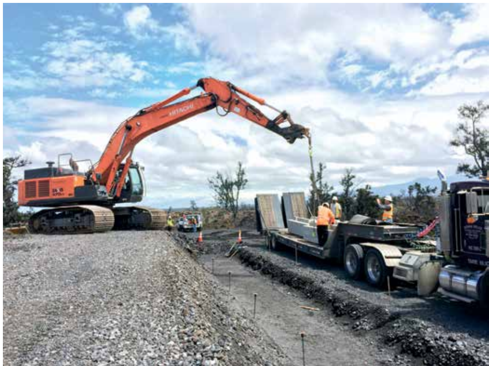
Goodfellow Bros.’ work at the Pohakuloa Training Area PHOTO COURTESY GOODFELLOW BROS.
