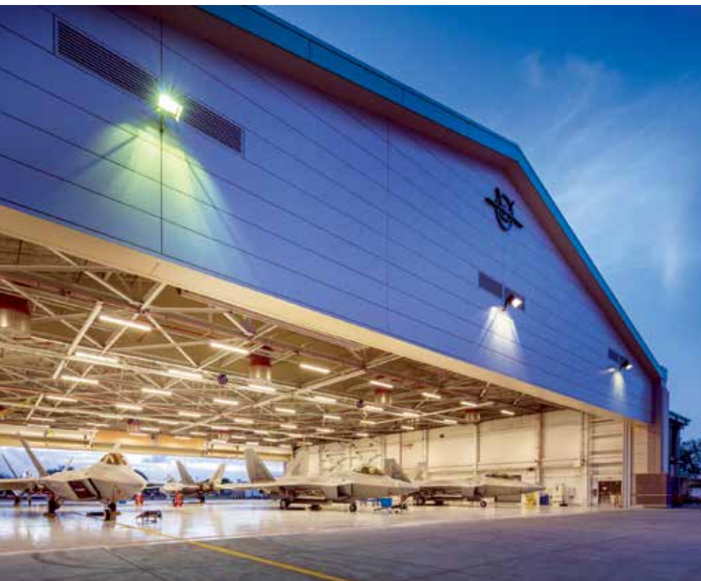
F-22 Raptors in the Daniel K. Inouye hangar built by Watts Constructors PHOTO COURTESY WATTS CONSTRUCTORS LLC
