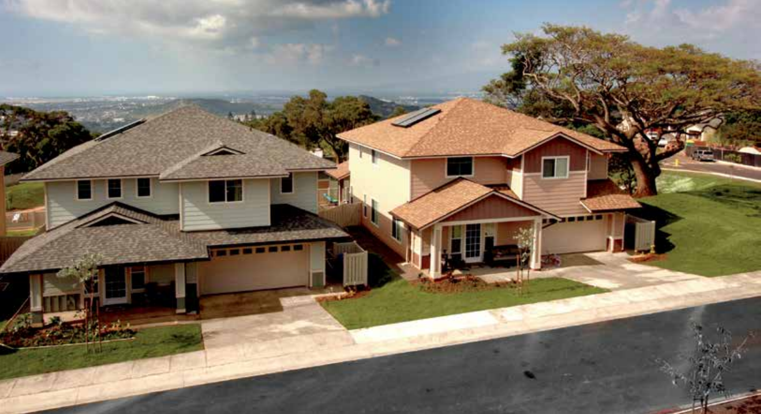
Lend Lease Hawaii completed Rainbow Village above Tripler Army Hospital in March. PHOTO COURTESY LEND LEASE HAWAII
