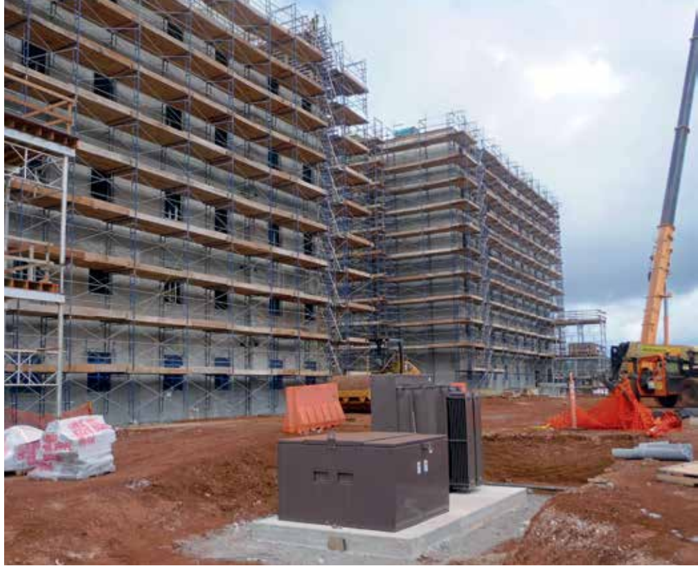
Nan Inc.'s twin six-story CAB barracks are aiming for LEED Silver certification. PHOTO COURTESY NAN INC.
