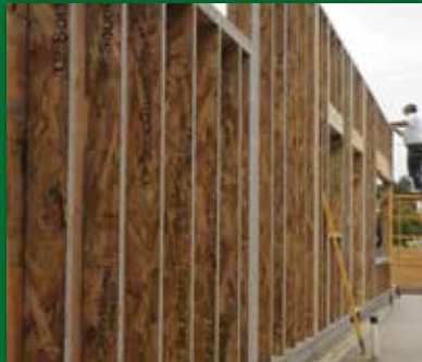
LSL WALL PANELS @ HOSPICE, KAMUELA
