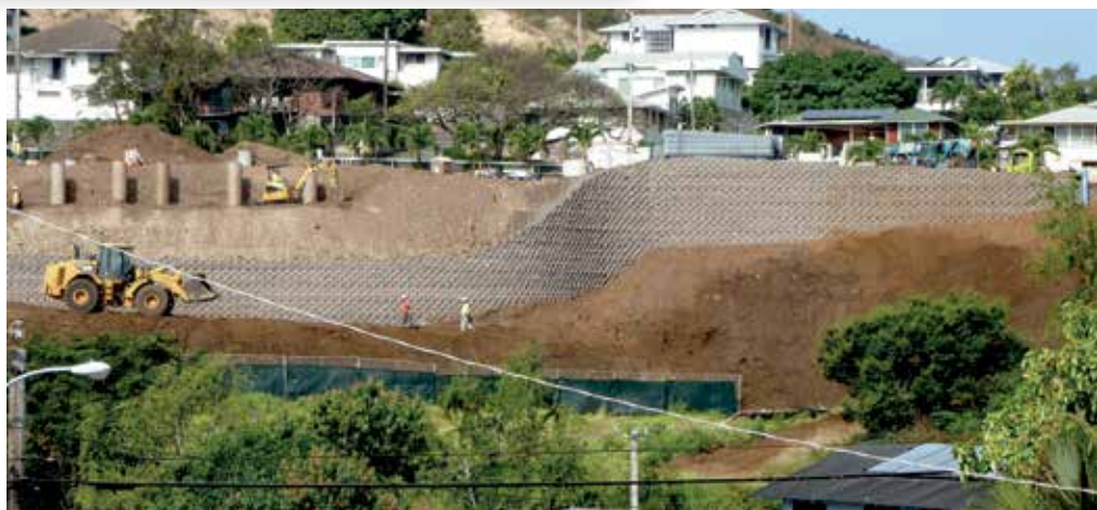
Nan Inc. constructs earthworks and a retaining wall on the slopes of Punchbowl. PHOTO COURTESY NAN INC./MICHAEL HEW
