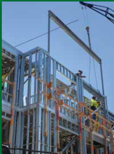
STEEL FRAMING @ KA MALANAI, KAILUA
