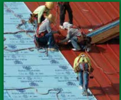
CUSTOM METAL ROOFING
