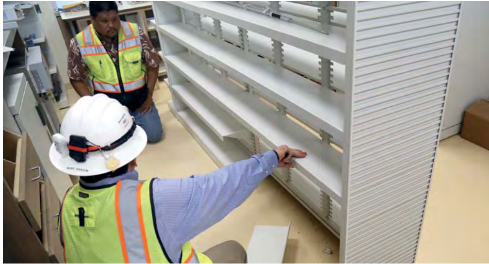
Robert Tomas of Hawaiian Dredging (top) and Michael Okamoto of Next Design during installation of OFVI (Owner Furnished Vendor Installed) shelving
