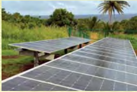
Haleakala National Park Off Grid PV System
