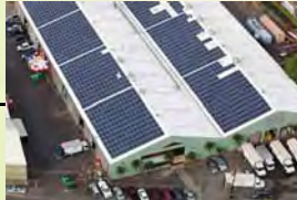
United Laundry, Plant Operations Roofing & PV Installation
