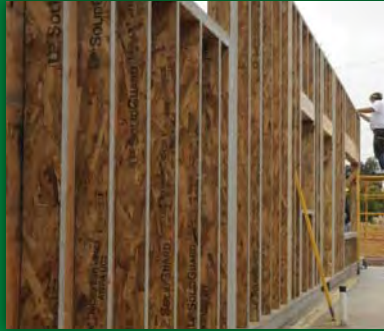
LSL WALL PANELS @ HOSPICE, KAMUELA
