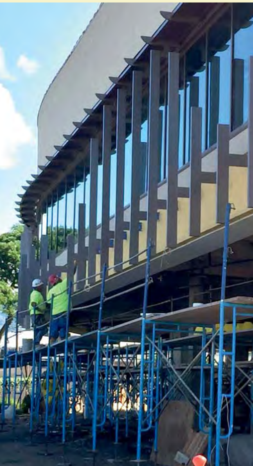
Construction of the new PBS Hawaii shows the light shelf and the supports for the bris soleil, two of the property's green features.
