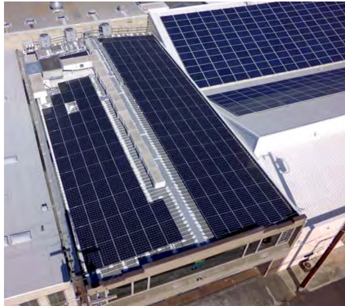
A Hi-Power Solar commercial PV project
