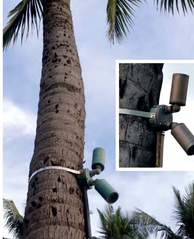
Outdoor lighting is popular throughout the Islands.
