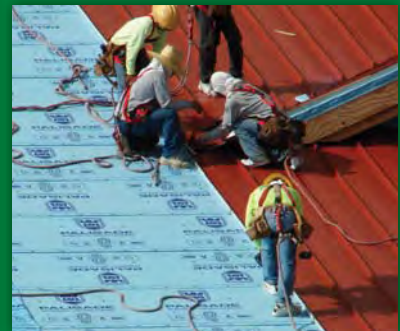
CUSTOM METAL ROOFING
