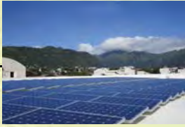
Japanese Cultural Center of Hawai'i, Roofing & PV Installation
