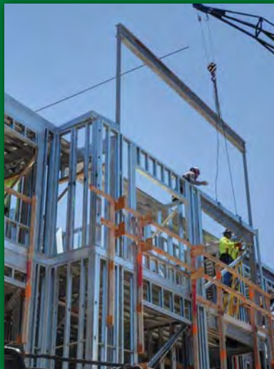
STEEL FRAMING @ KA MALANAI, KAILUA
