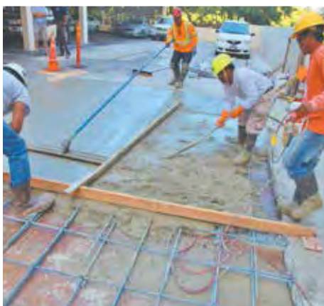
PARKING DECK & PT CABLE REPAIRS
