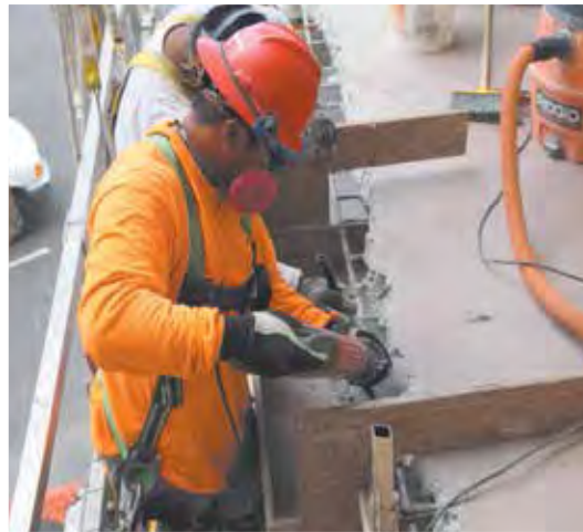
HIGH-RISE SPALL REPAIR
