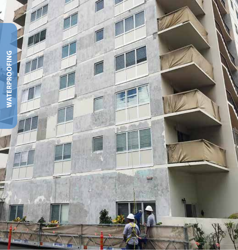
The exterior of a building is stripped to bare concrete after it was determined that the building could not receive any more coating until all of the existing paint was completely removed. The building then was given a new system of one coat of primer, one coat of elastomeric and two topcoats of 100 percent acrylic.
