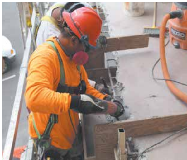
HIGH-RISE SPALL REPAIR
