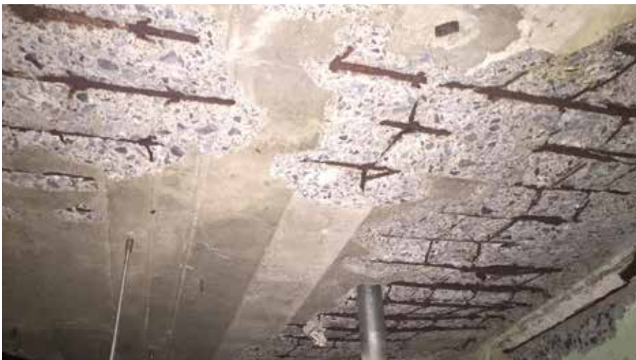
Spalled concrete is expanded corroded steel which causes the concrete to fall away from the structure.
