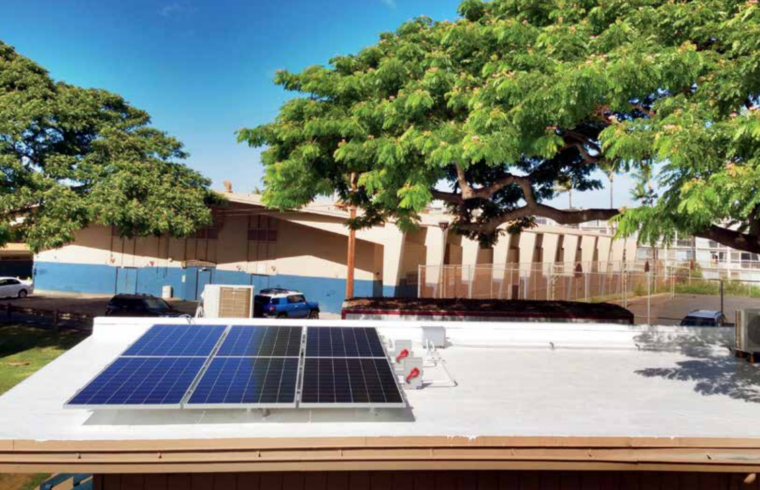
Two hybrid solar ACs were installed as a pilot project out at Waianae High School to reduce the heat in one of the hottest portables on campus.
