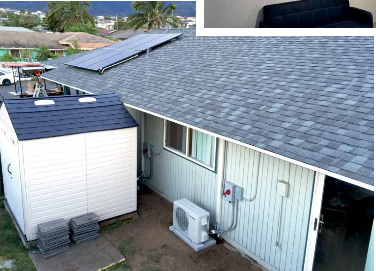
Outside PV and condenser units with indoor wall mounted-evaporators. Inside, the house has a standard ductless split system AC.
