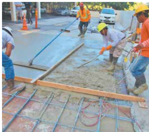
PARKING DECK & PT CABLE REPAIRS
