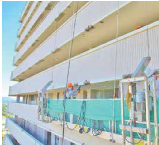
HIGH-RISE SPALL REPAIR
