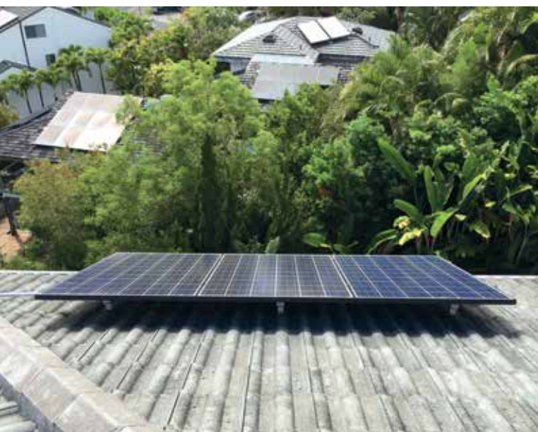
Minimal footprint of 3 PV modules feed directly into the Hybrid A/C. No utility feedback. No wait times.
