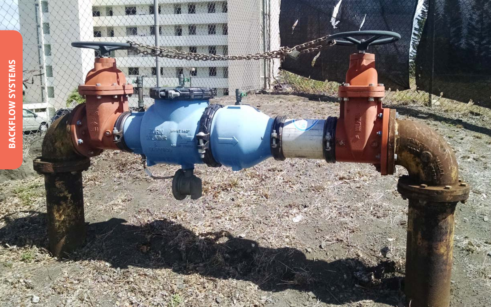
An above-ground backflow system commonly used in Hawaii
