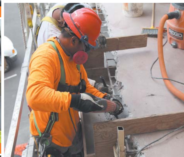
HIGH-RISE SPALL REPAIR
