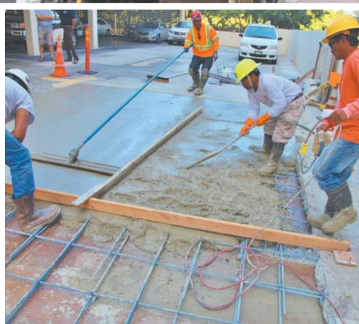
PARKING DECK & PT CABLE REPAIRS
