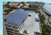
AOAO 215 N. King Street Solar PV Carport Installed
