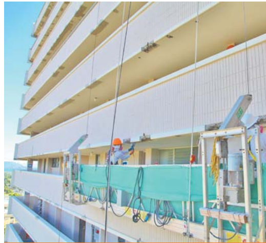
HIGH-RISE SPALL REPAIR
