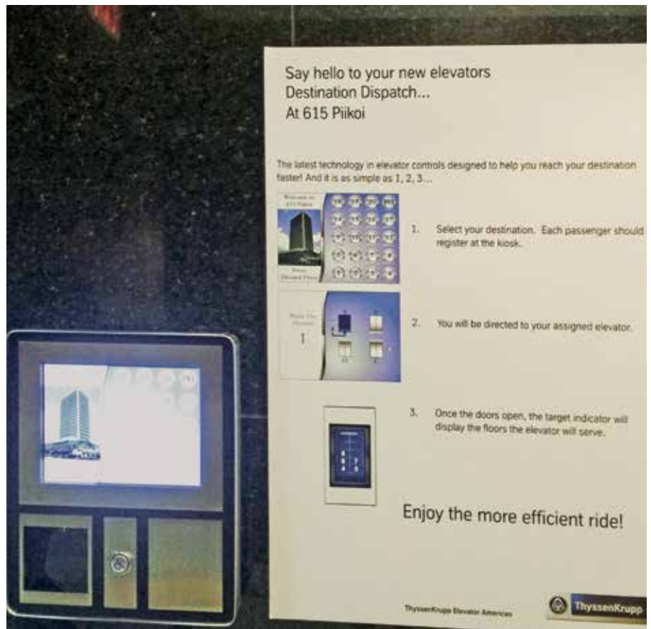
This touch-screen, destination dispatch kiosk directs people to an assigned elevator, cutting travel time.
