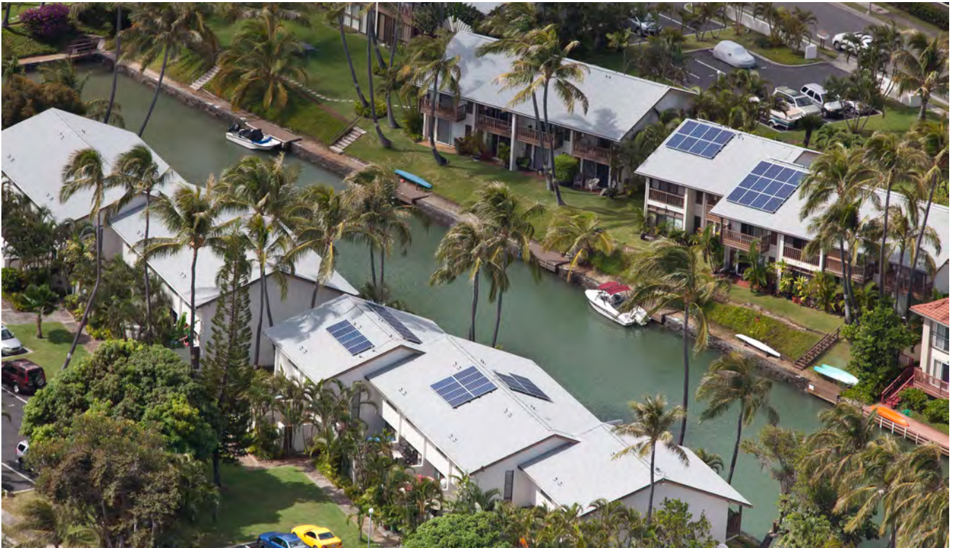
CRW installed CertainTeed shingles at this Hawaii Kai complex.
