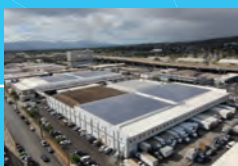
Unicold Cold Storage Facilities Solar Roofing Installation
